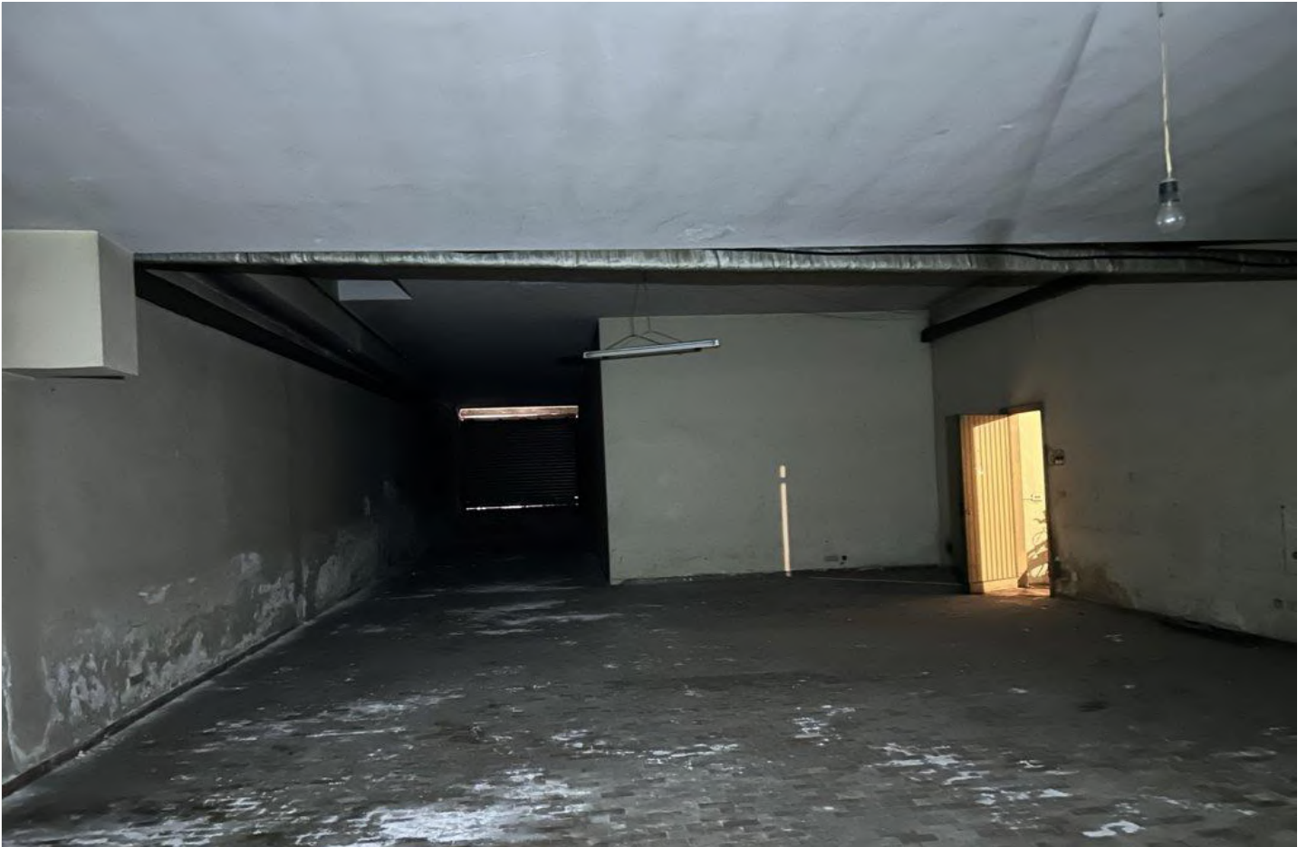
Sub. 25 - interno garage piano seminterrato
