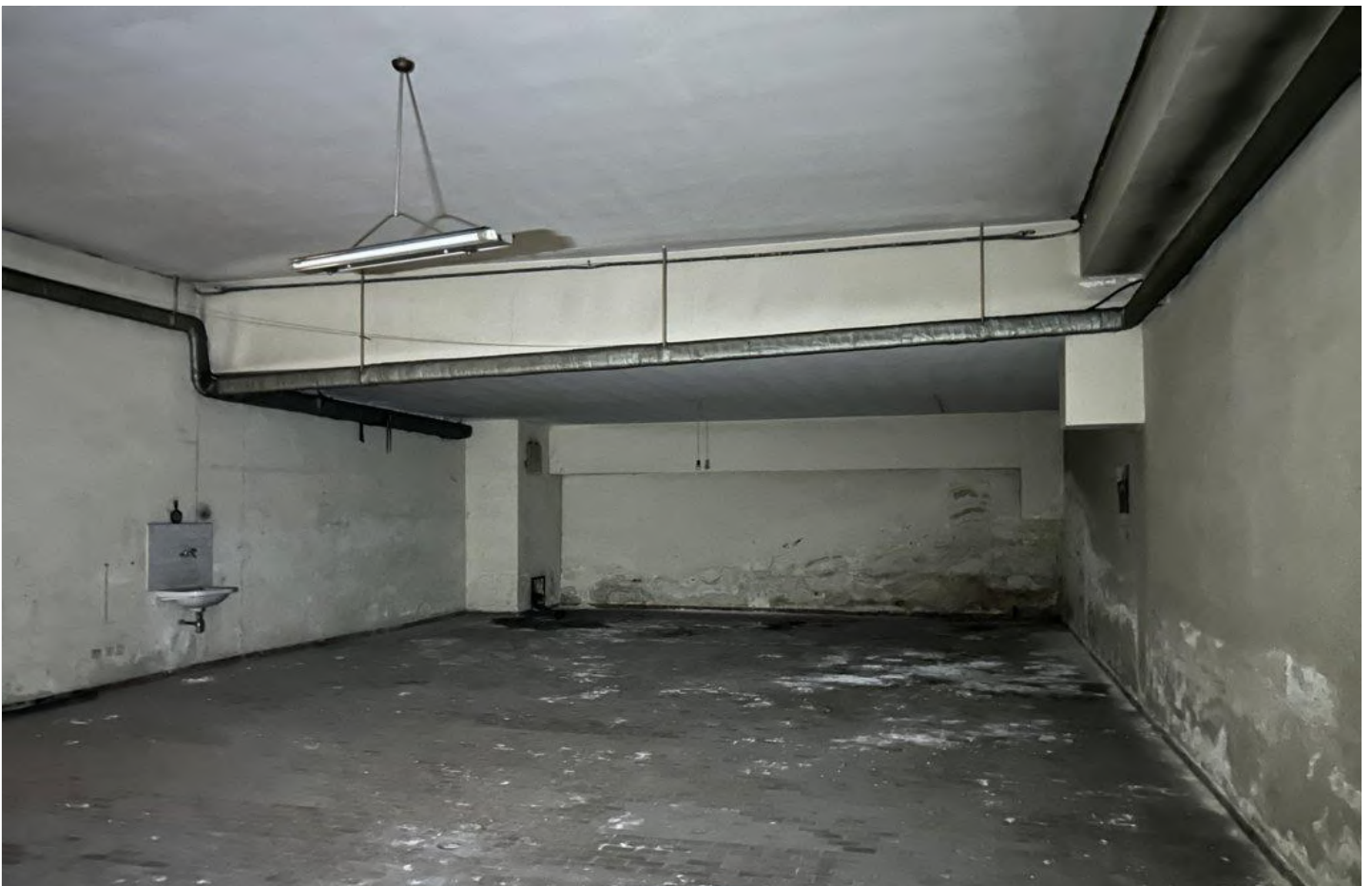
Sub. 25 - interno garage piano seminterrato
