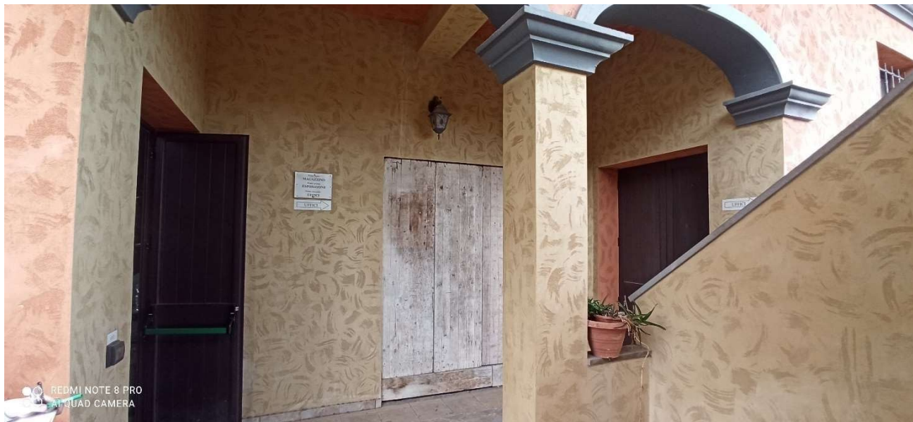
vista accessi a piano terra – sx sub.8, dx sub.9
