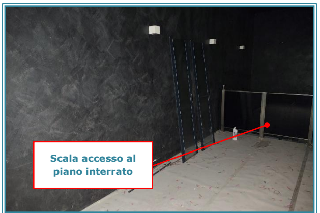
Figura 25 Sala1 – Piano Terra
