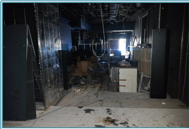
Figura 22 Sala1 – Piano Terra
