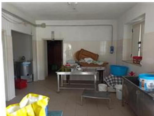
piano terra - laboratorio
