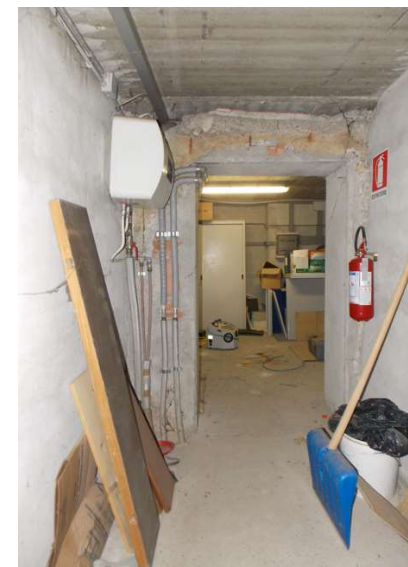
19A - corridoio piano interrato
