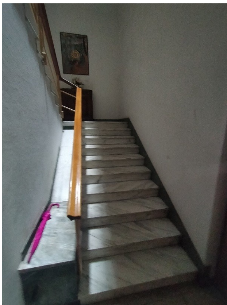
- RAMPE SCALE CONDOMINIALI -
