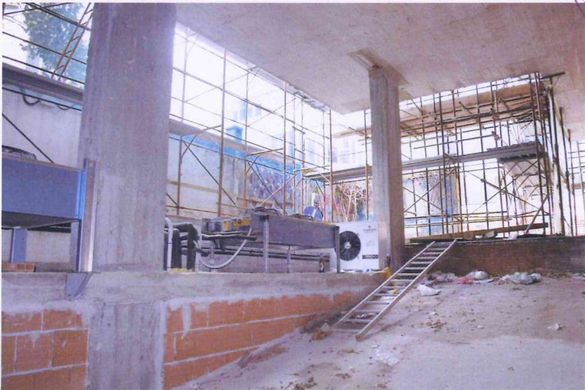
12. Controcampo rampa garages.
