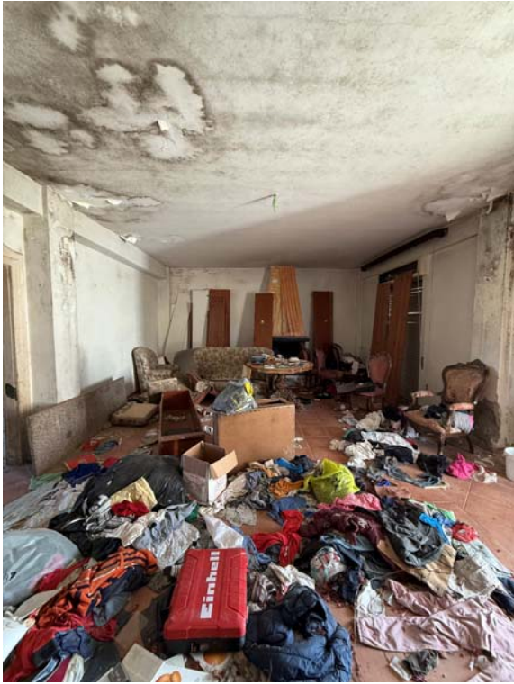
Salotto al piano terra (villa p.lla 256, sub. 1)
