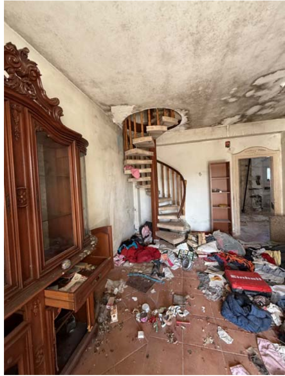
Salotto al piano terra (villa p.lla 256, sub. 1)
