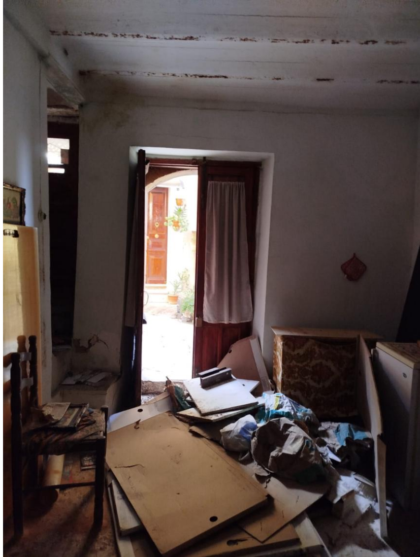
Foto 4 – piano terra (foglio 130 particella 1911 sub. 1)
