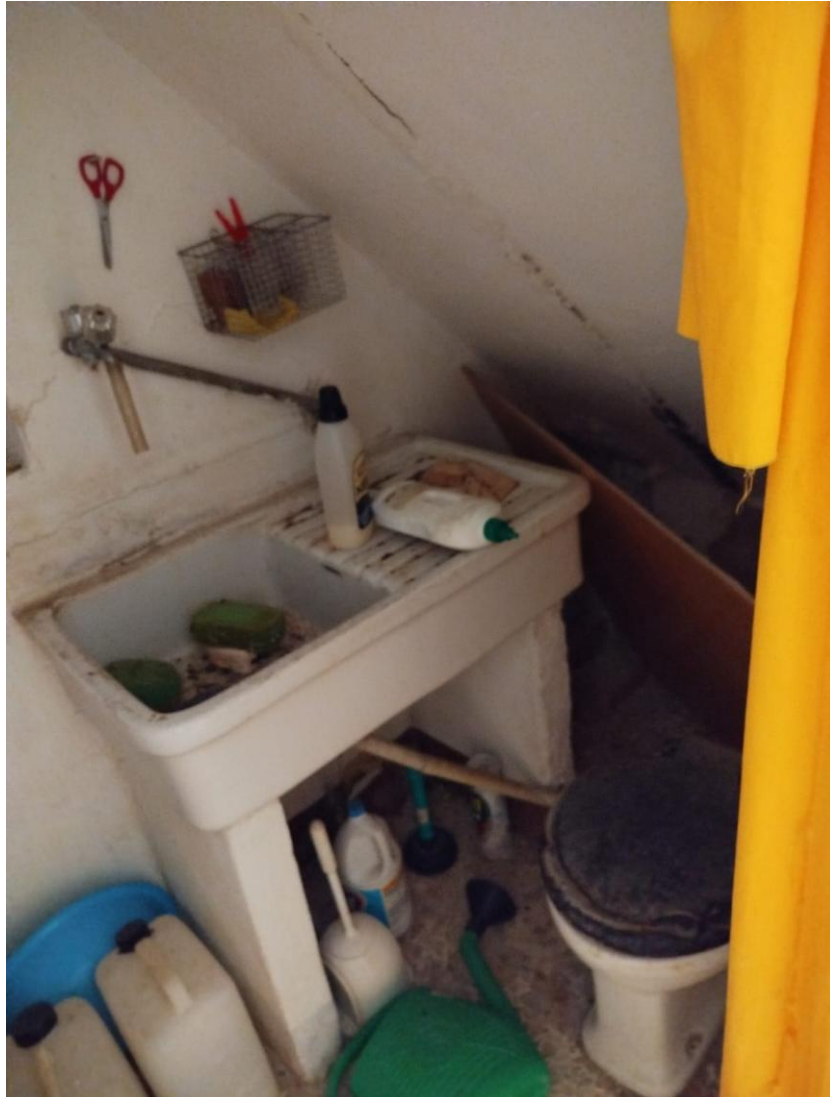
Foto 6 – piano terra- wc (foglio 130 particella 1911 sub. 1)
