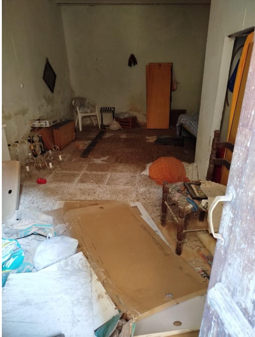
Foto 5 – piano terra (foglio 130 particella 1911 sub. 1)
