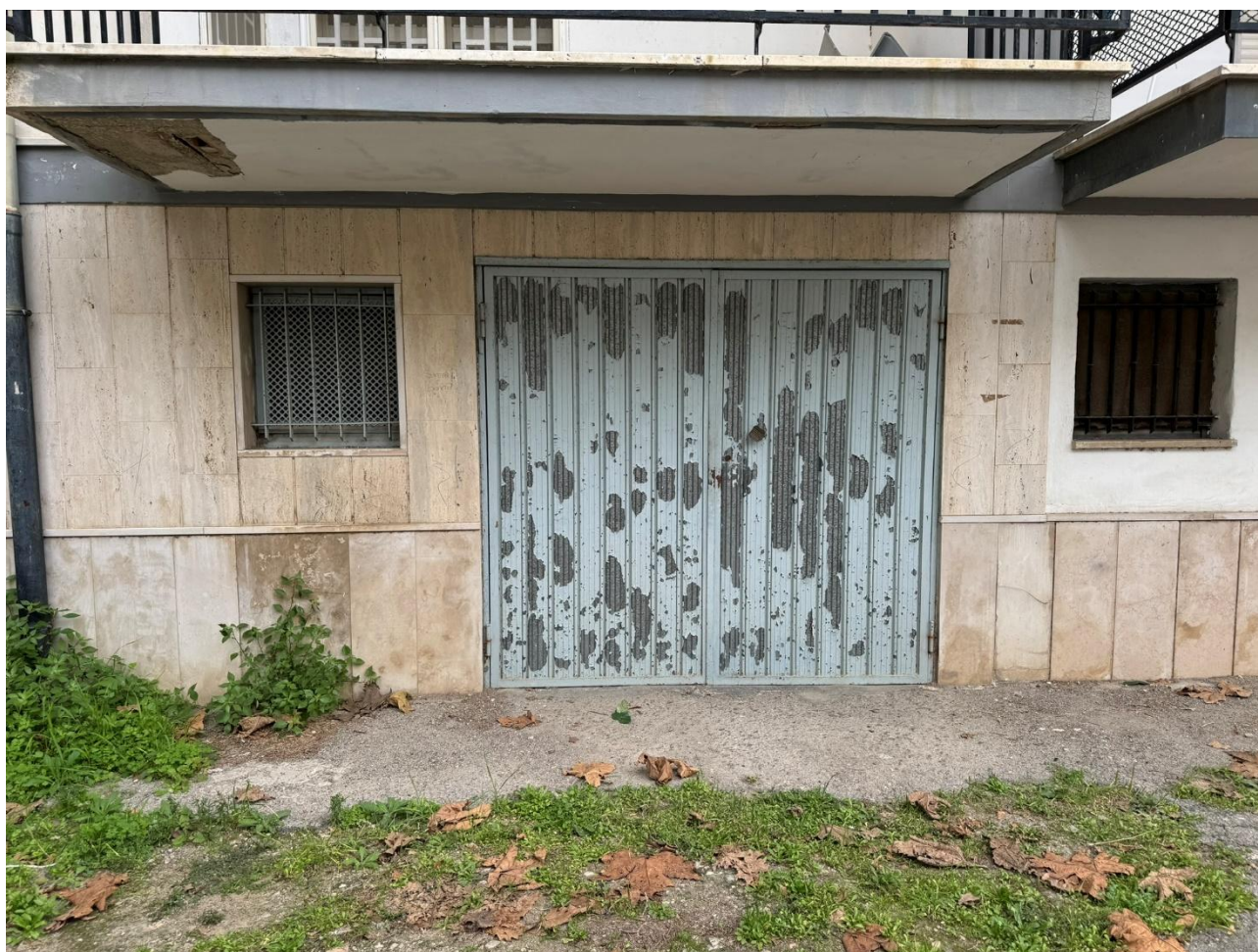
CANTINOLA IN PIANO TERRA
