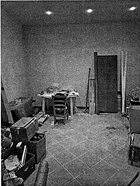
Locale piano terra
