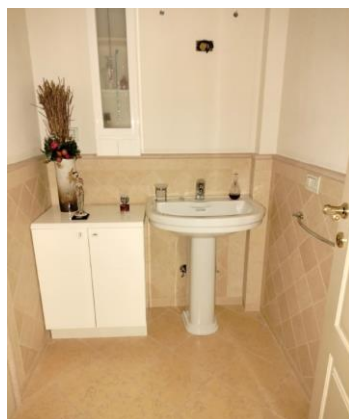
Bagno piano seminterrato
