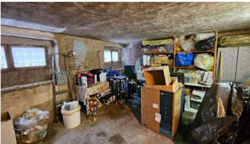
Cantina piano seminterrato
