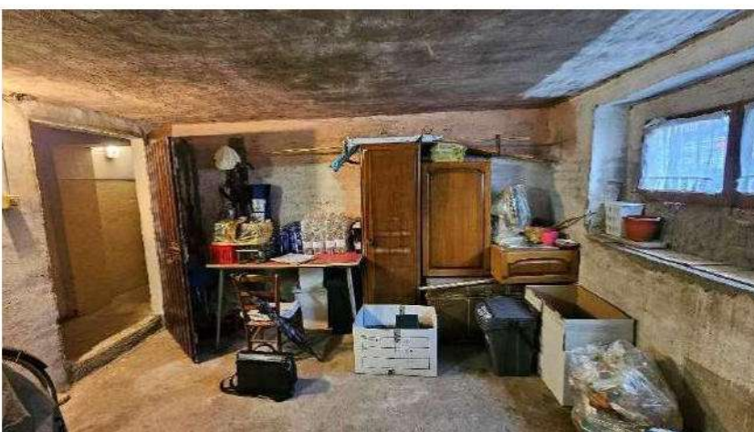
Cantina piano seminterrato
