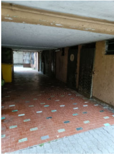
Cantine a piano terreno
