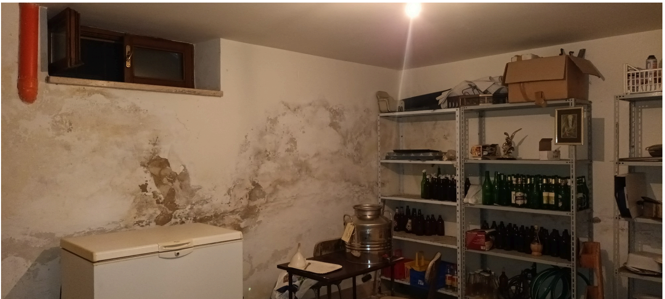
Piano seminterrato – cantina
