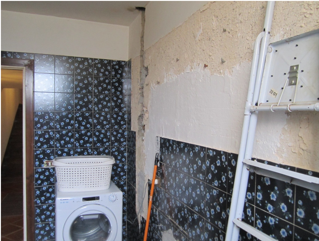
Bagno piano interrato
