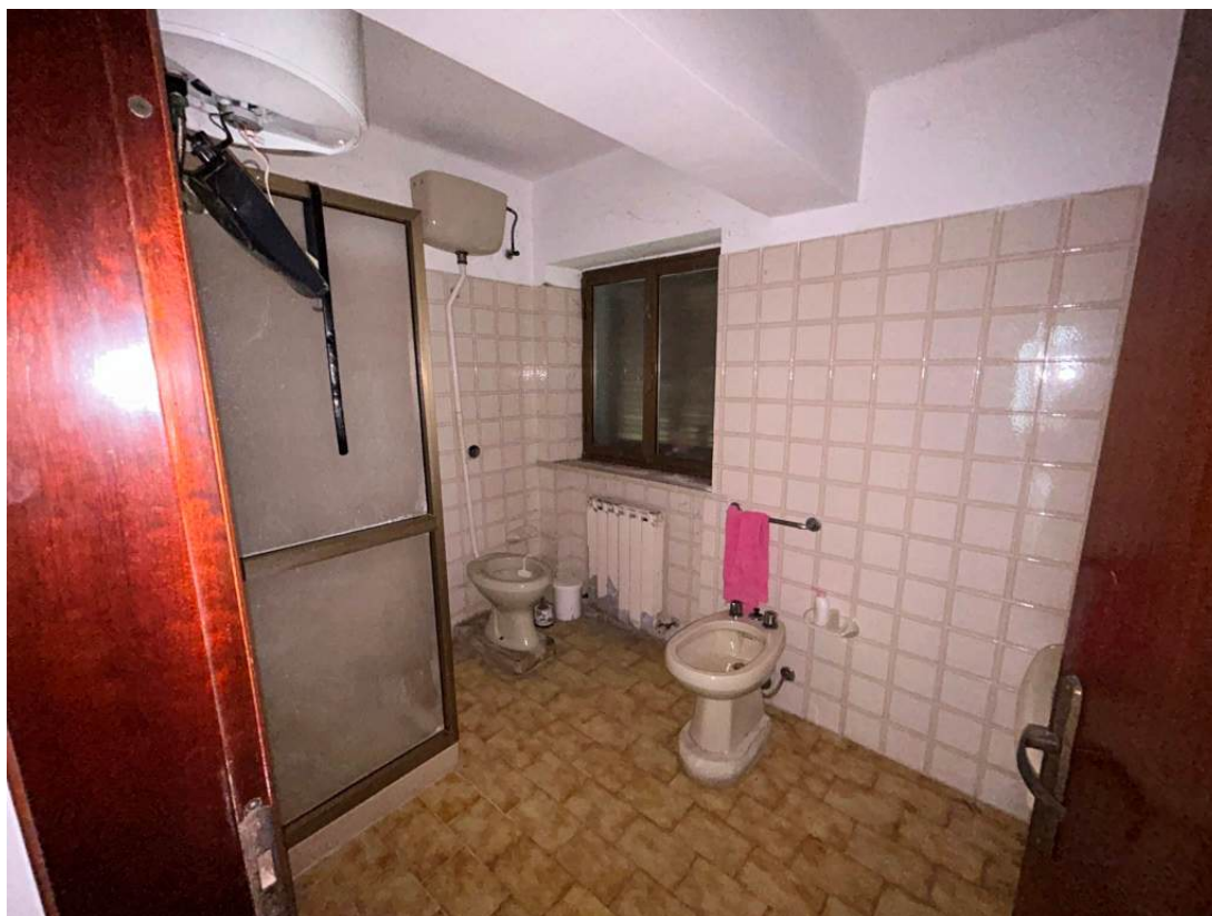
BAGNO (w.c.) – Piano Terra – vista 1
