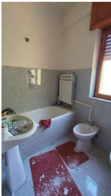
Figura 21: wc piano terra
