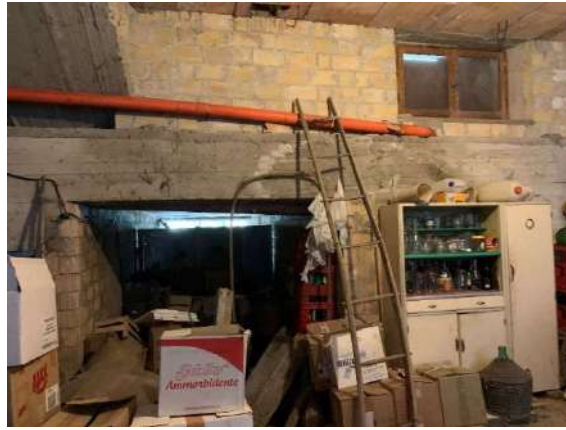
GARAGE PART. 279 SUB 3
