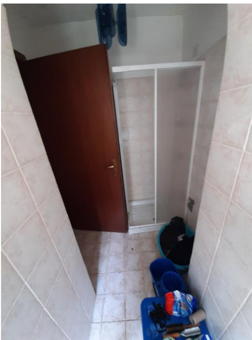
Bagno piano terra
