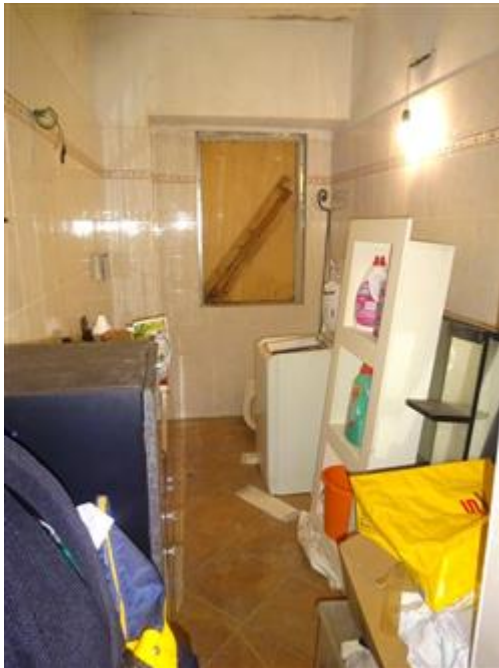
Bagno piano terra
