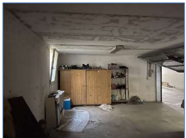
12. Piano interrato - Garage
