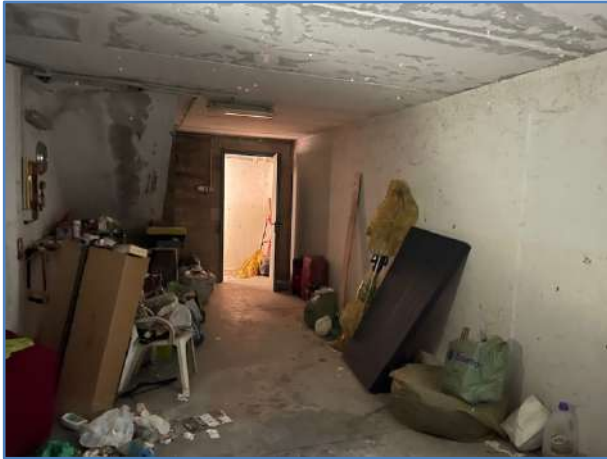
13. Piano interrato - Garage
