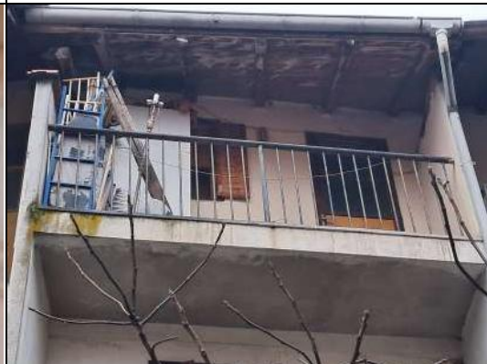
▲ Vista locali 2 piano
