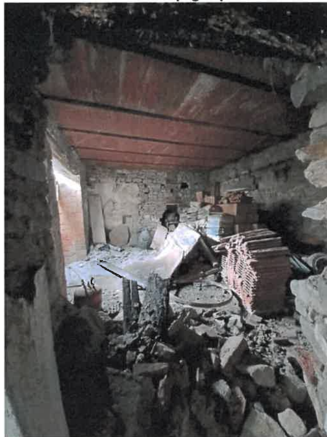
Vista interna - Camera piano terra
