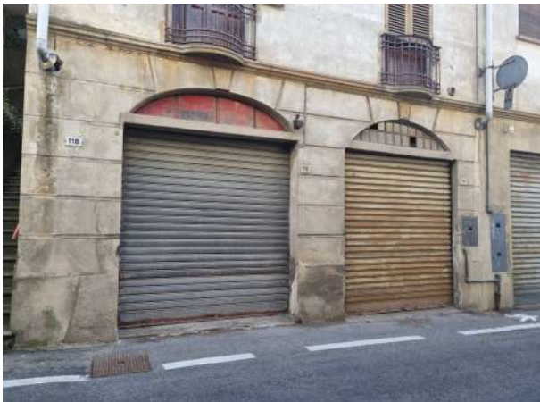
SERRANDE PIANO TERRENO
