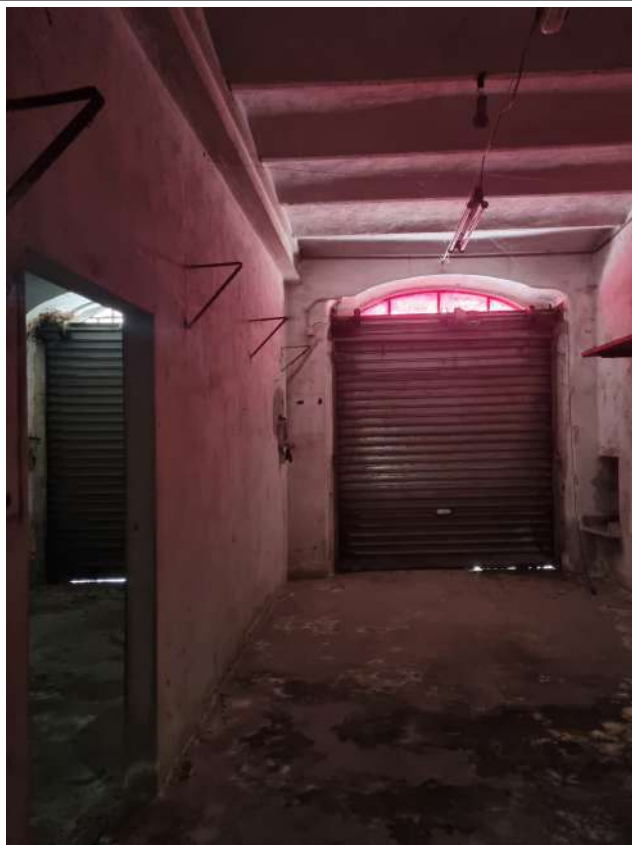
SERRANDA INTERNA PIANO TERRENO
