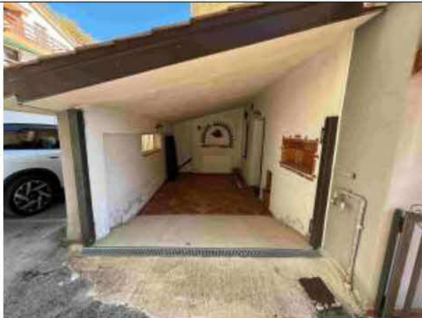
Piano terra- Vista box auto
