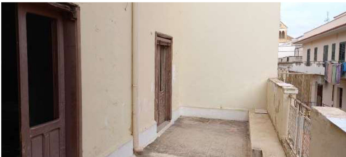
Foto 11 – Immobile “1A” – Balcone a I P
