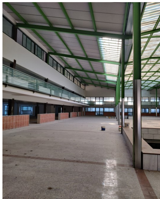
(Foto 8) – piano terra
