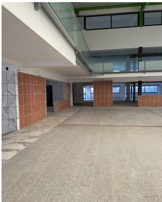
(Foto 7) – piano terra
