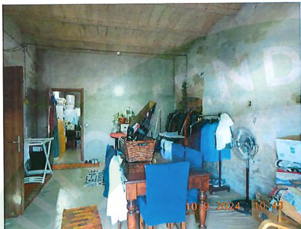
Sub 2 – piano terra – androne
