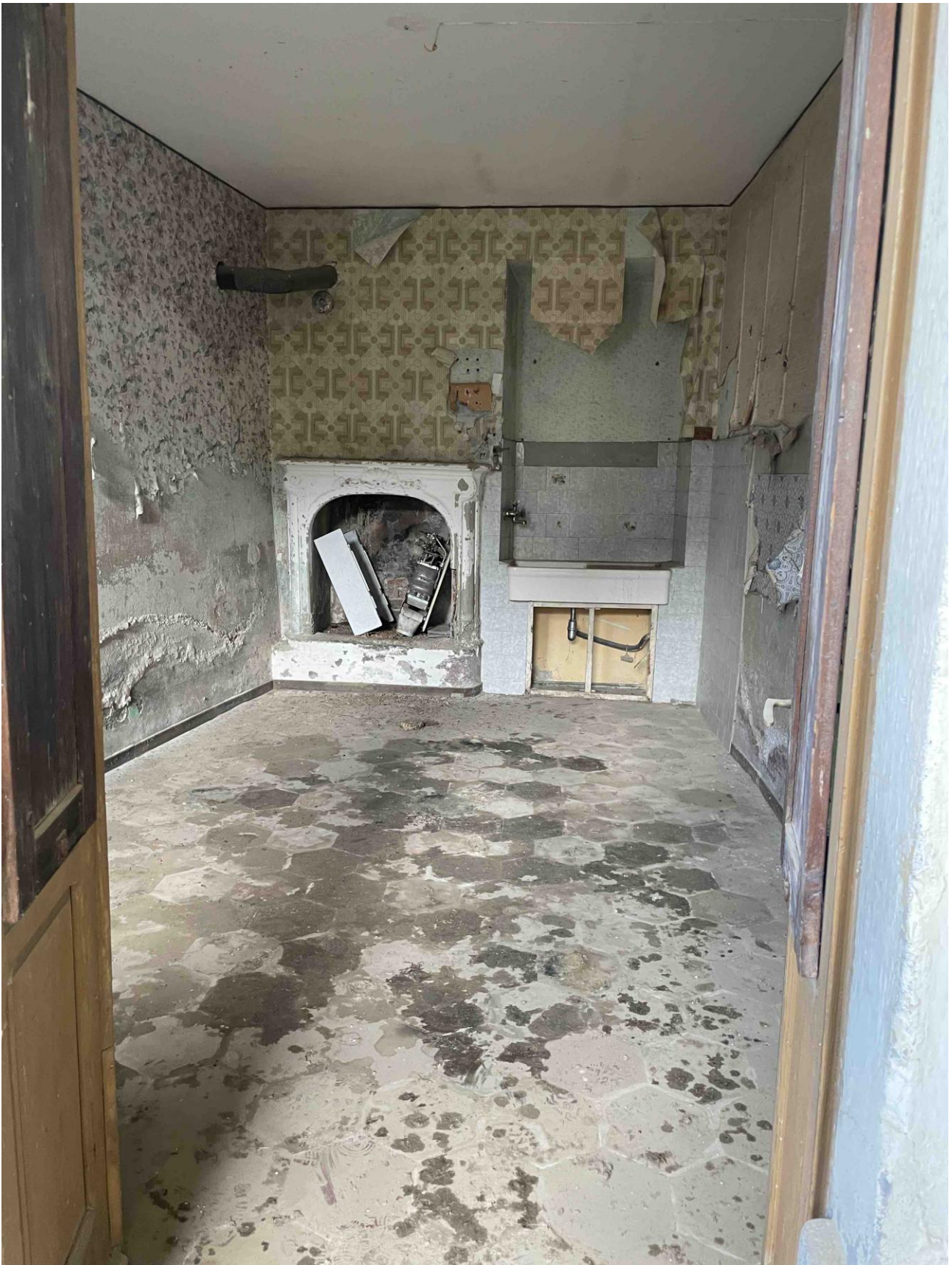
LOCALE PIANO TERRA
