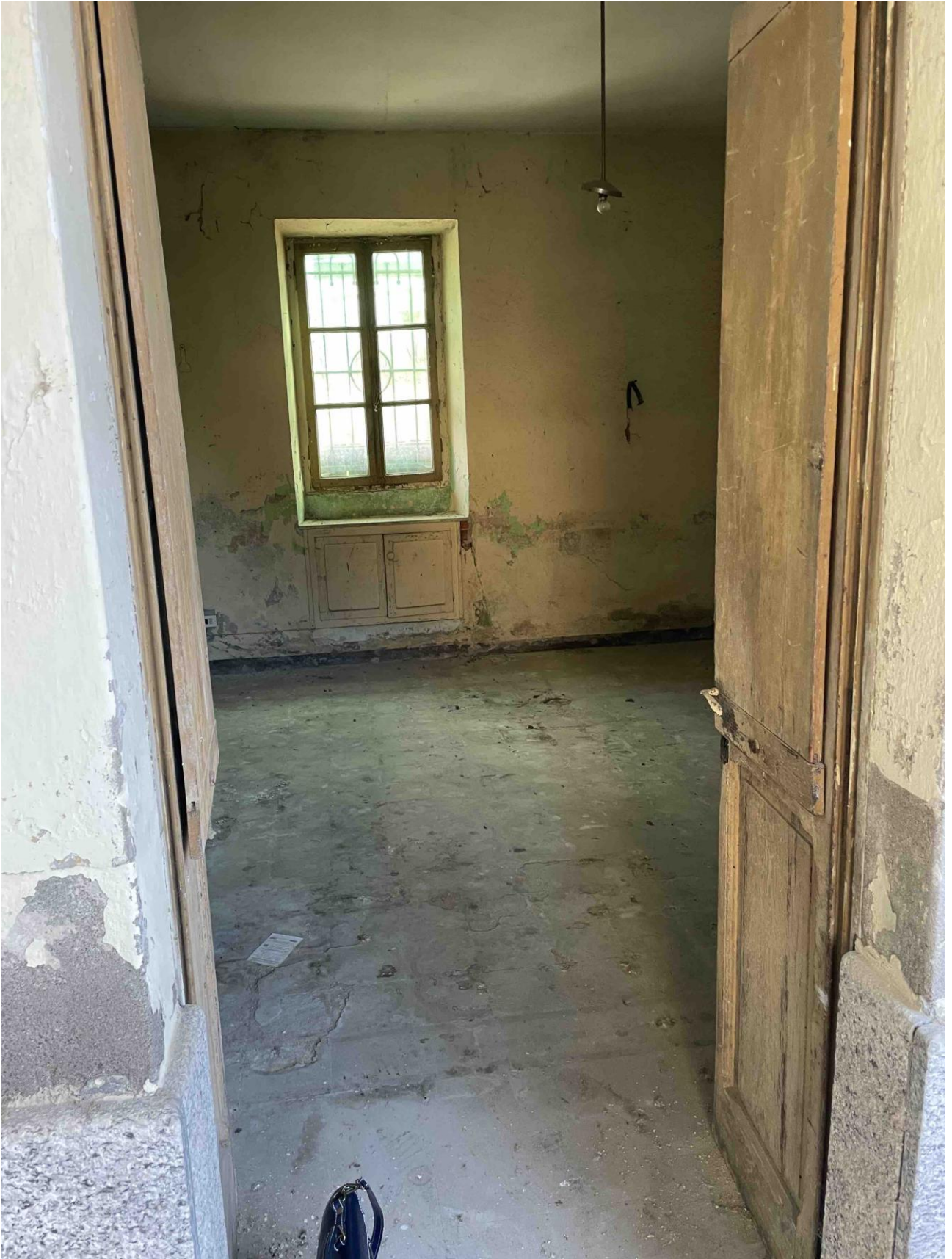
LOCALE SGOMBERO PIANO TERRA
