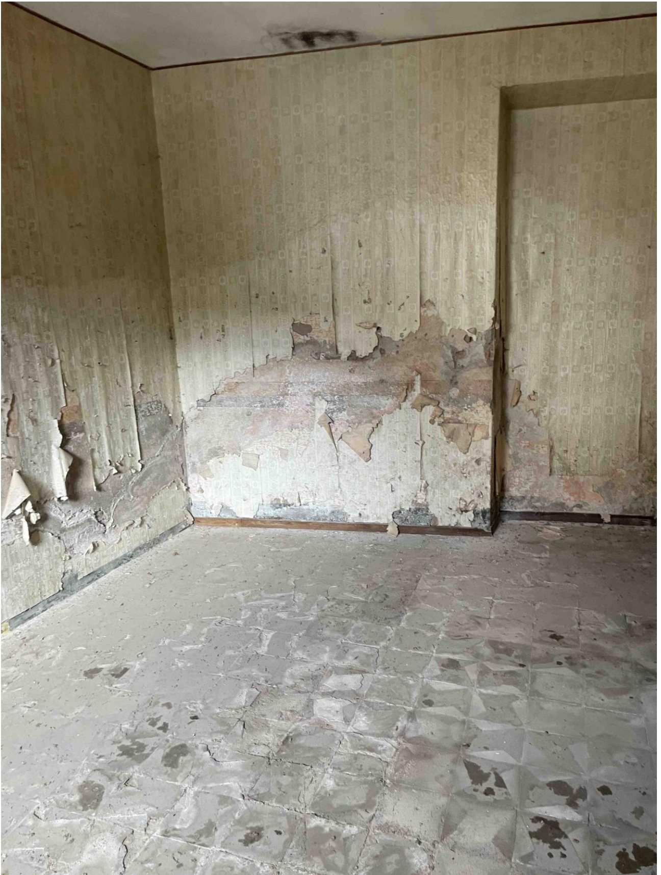
CAMERA PIANO TERRA
