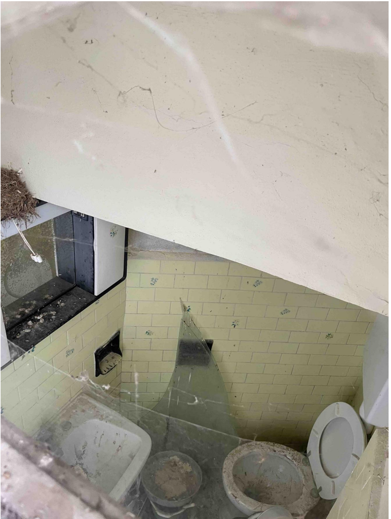
BAGNO PIANO TERRA
