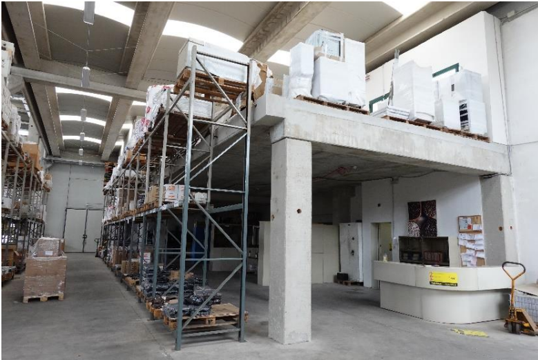
30 – area deposito open space e soppalco
