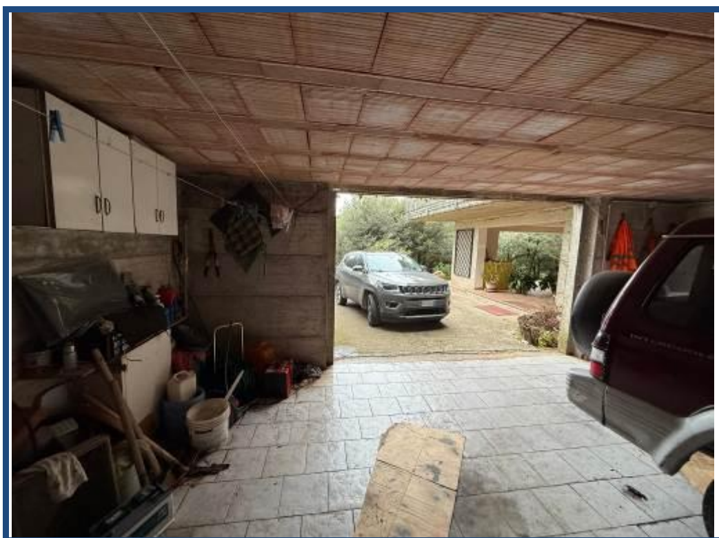
Foto 48 – Vista interna garage piano seminterrato – sub. 2
