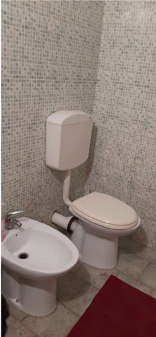
WC- Piano Interrato
