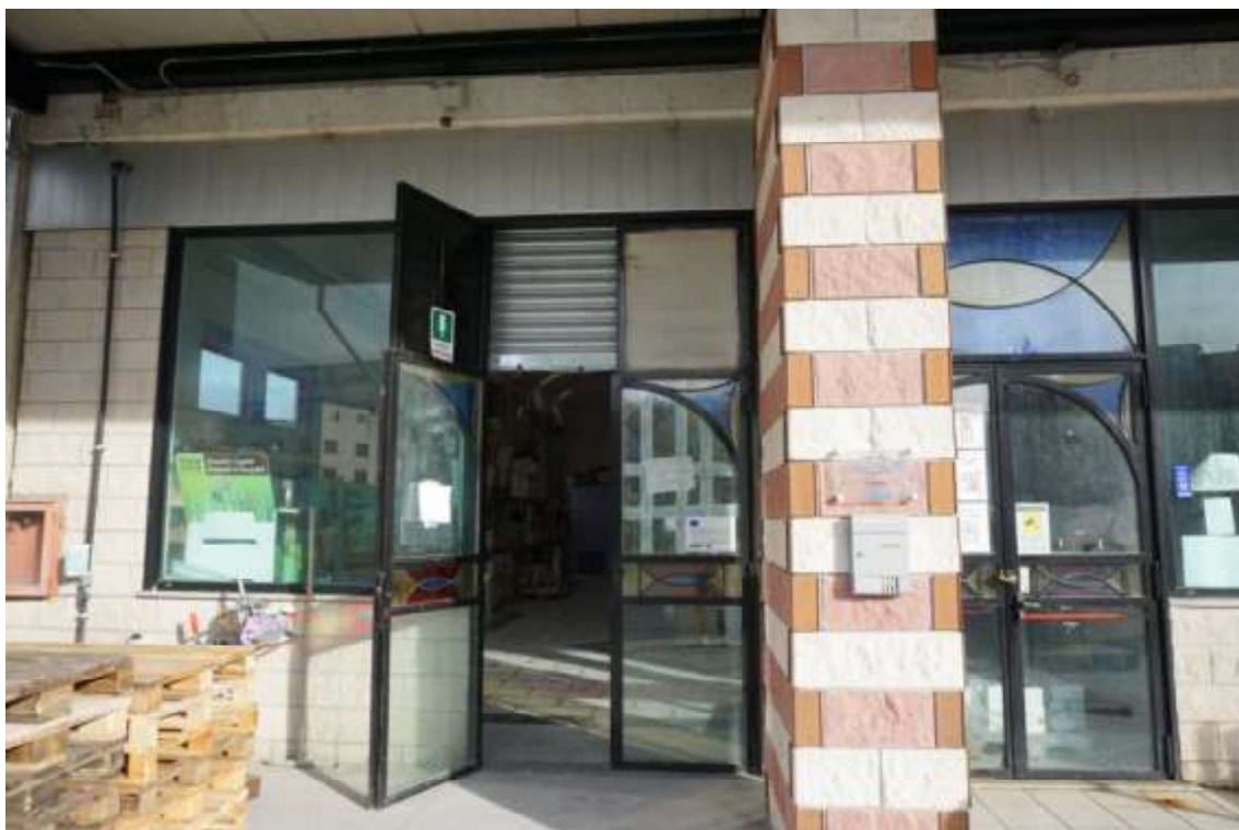
Fig.15 – Vista porte d’ingresso sub.18 (C1)
