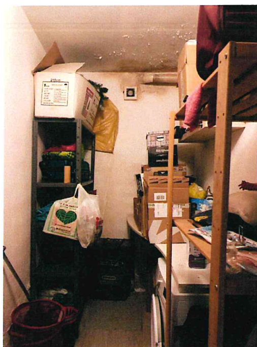
Locale cantina piano int.
