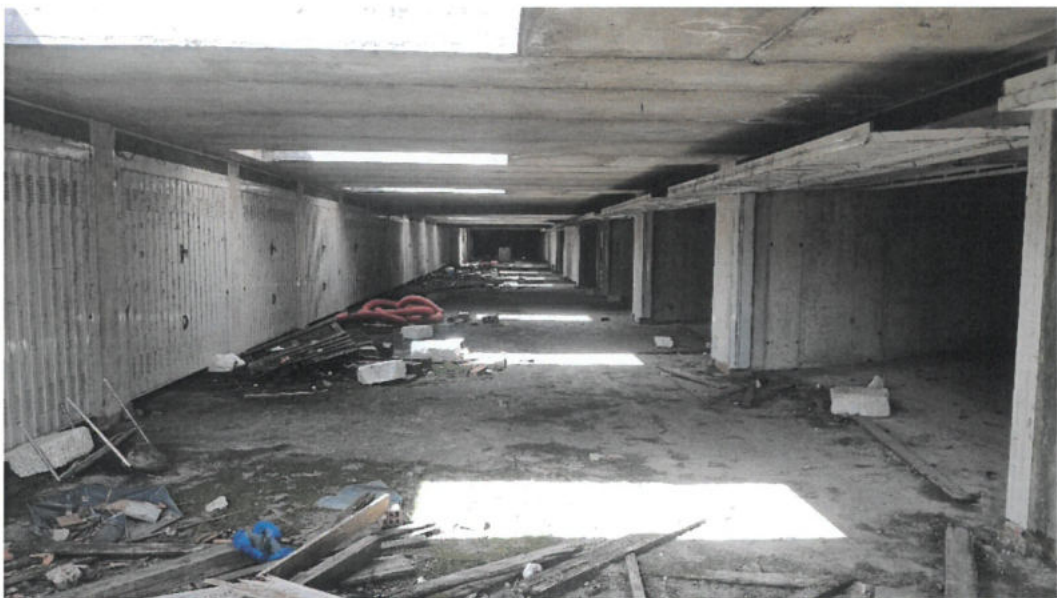
piano interrato - box
