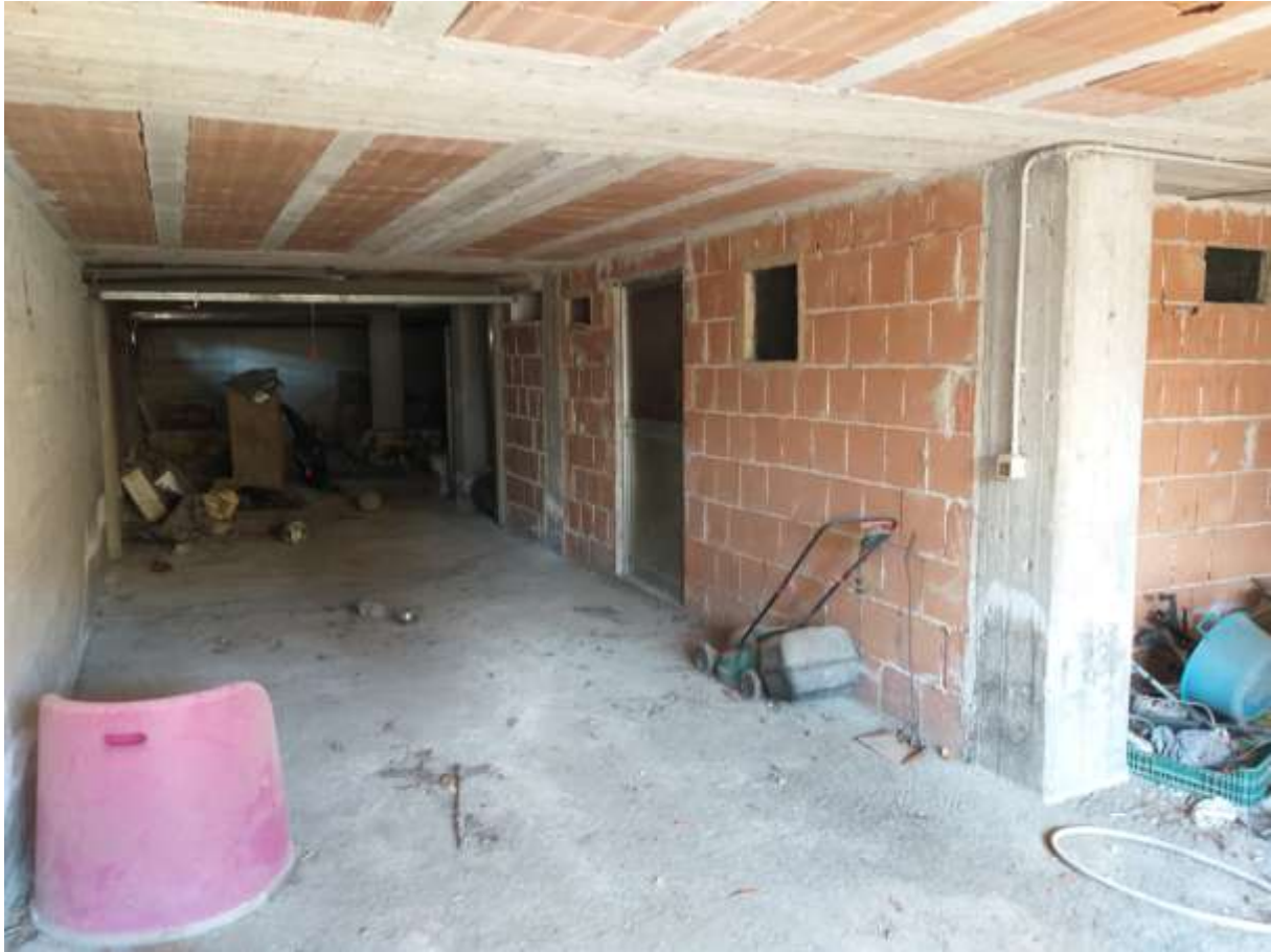
MAGAZZINO PIANO INTERRATO PART. 280 SUB. 2
