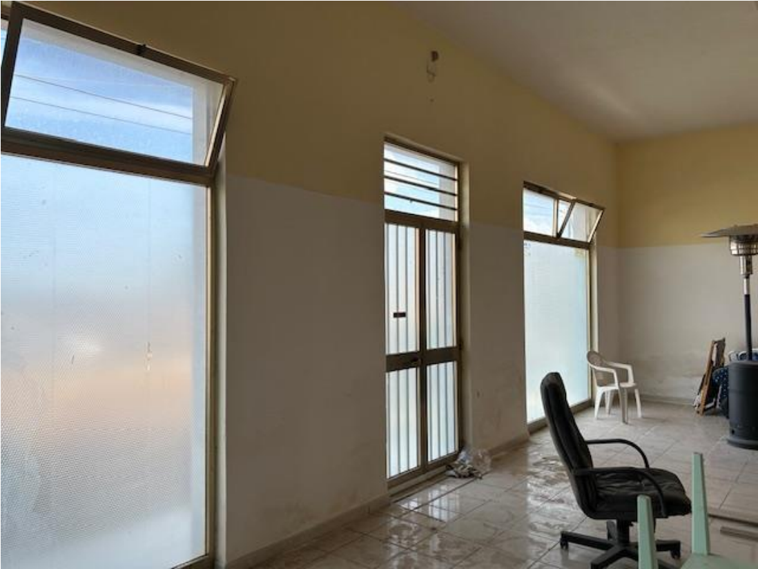
VISTE 4-5-6-7_Interni locale commerciale
