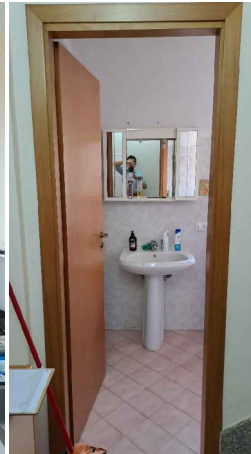
Bagno piano terra
