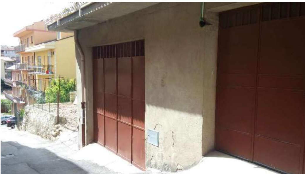
Foto 2 – esterno garage (foglio 14 particella 597 sub. 1 e 598 sub. 3)
