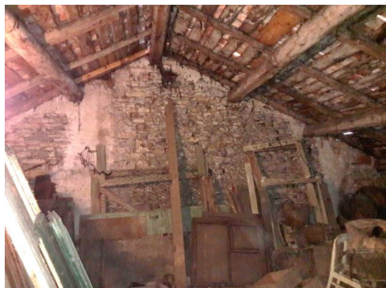
Part. 587 sub. 2 - P2 - Soffitta
