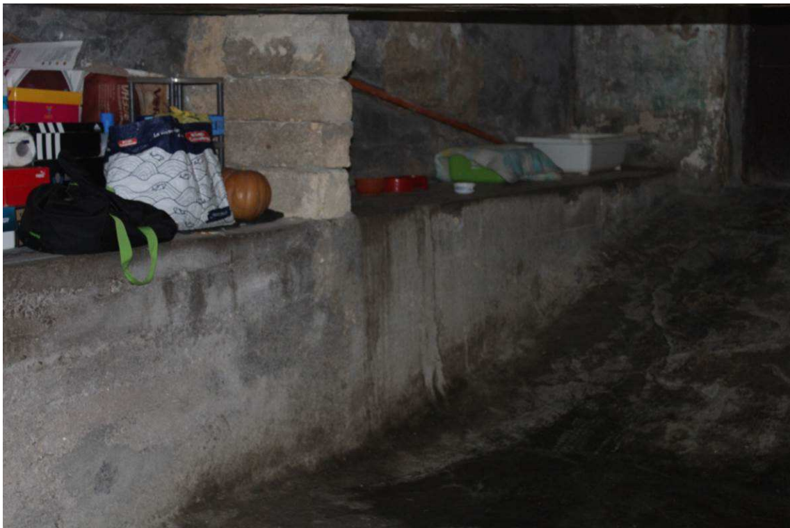
Piano seminterrato- cantina
