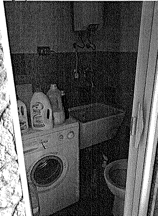
Bagno piano terra
