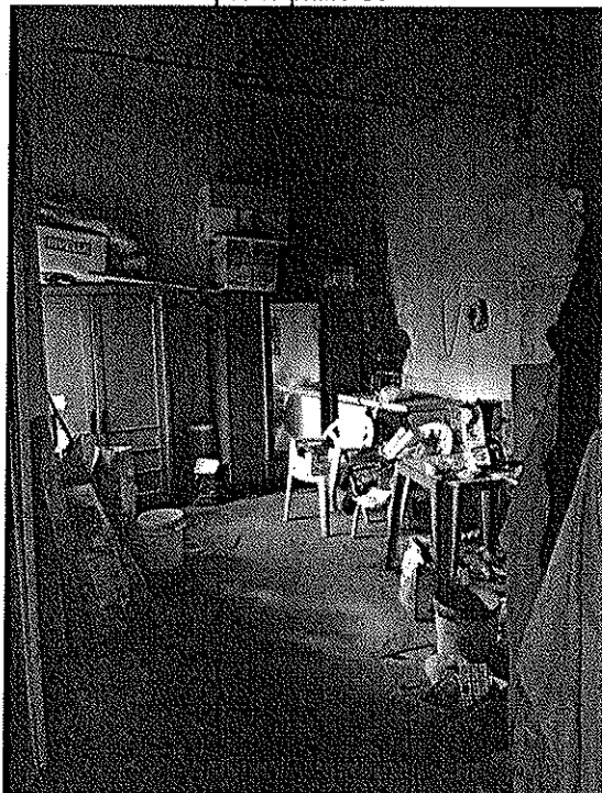
Interno locale deposito piano S1
