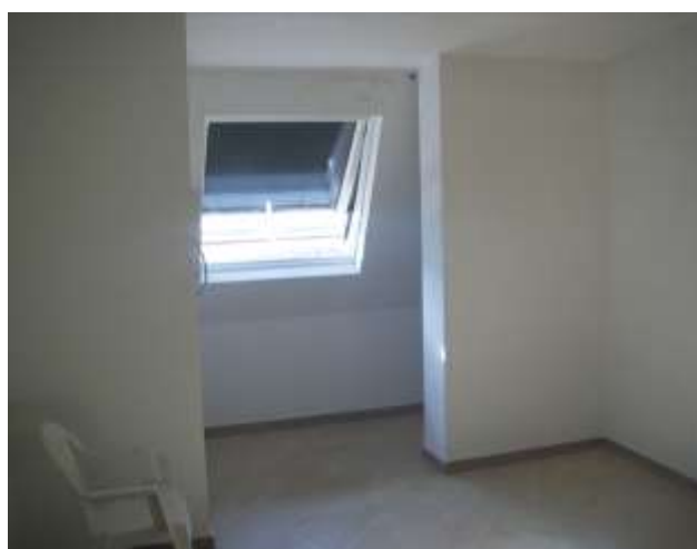
(foto 2: vista camera)
