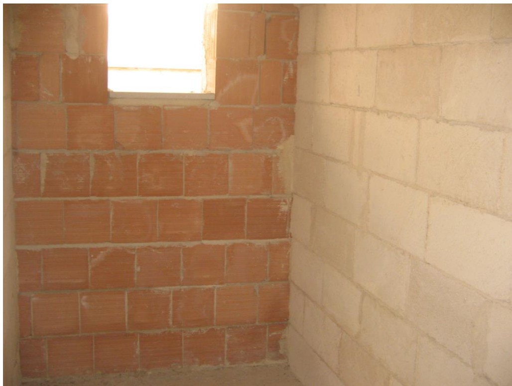
bagno – piano terra
