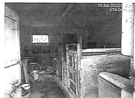
Figure 9- vista interna ex stalla
