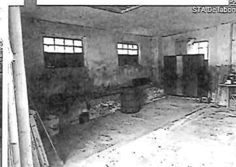
Figure 8- vista interna ex stalla
