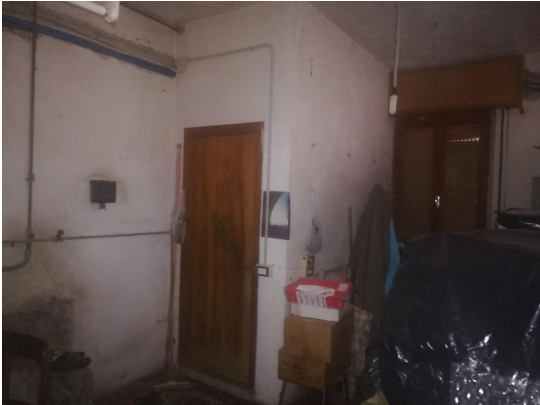
SUB. 24- PIANO TERRA : PORTA WC
