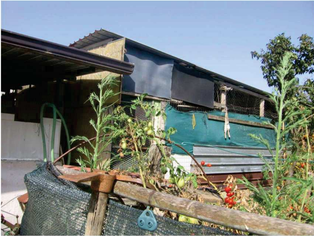
Strutture precarie abusive
