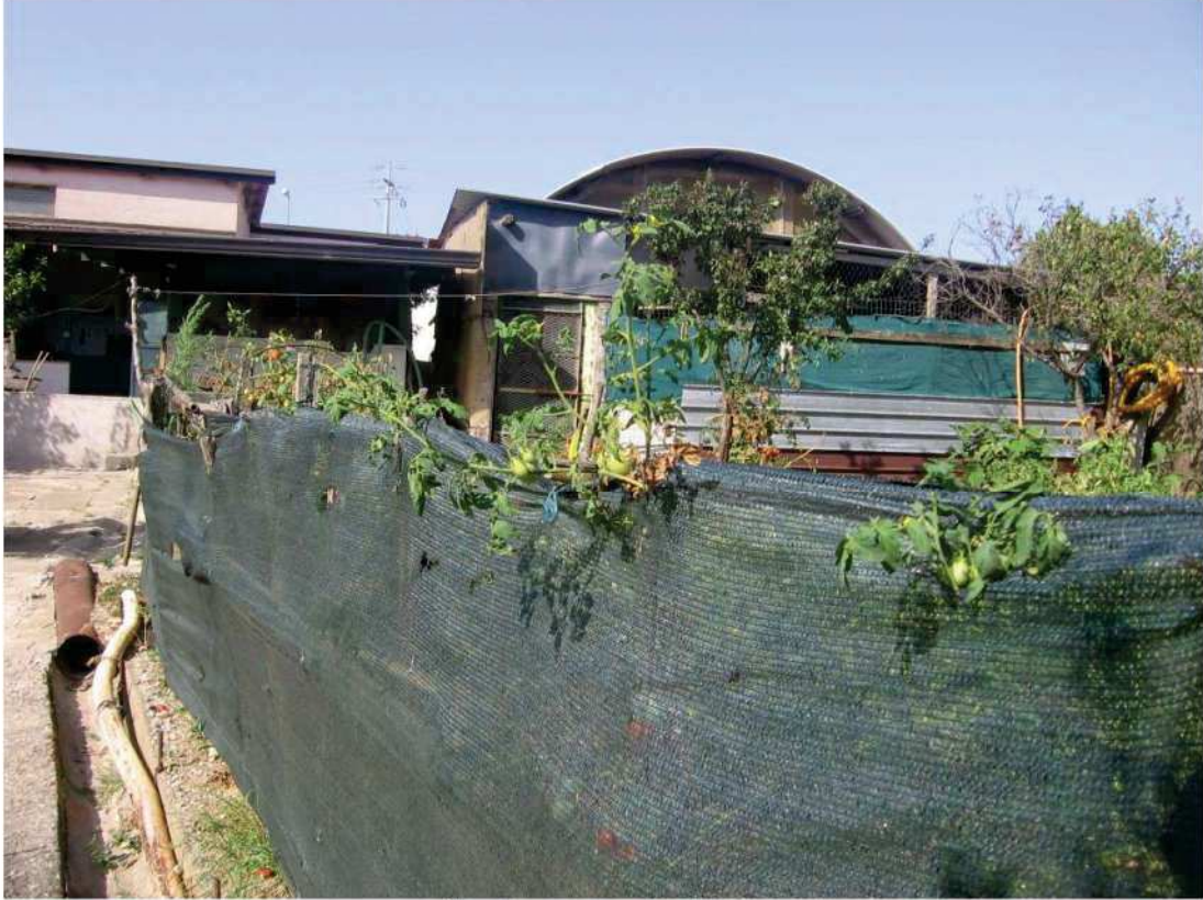
Strutture precarie abusive
