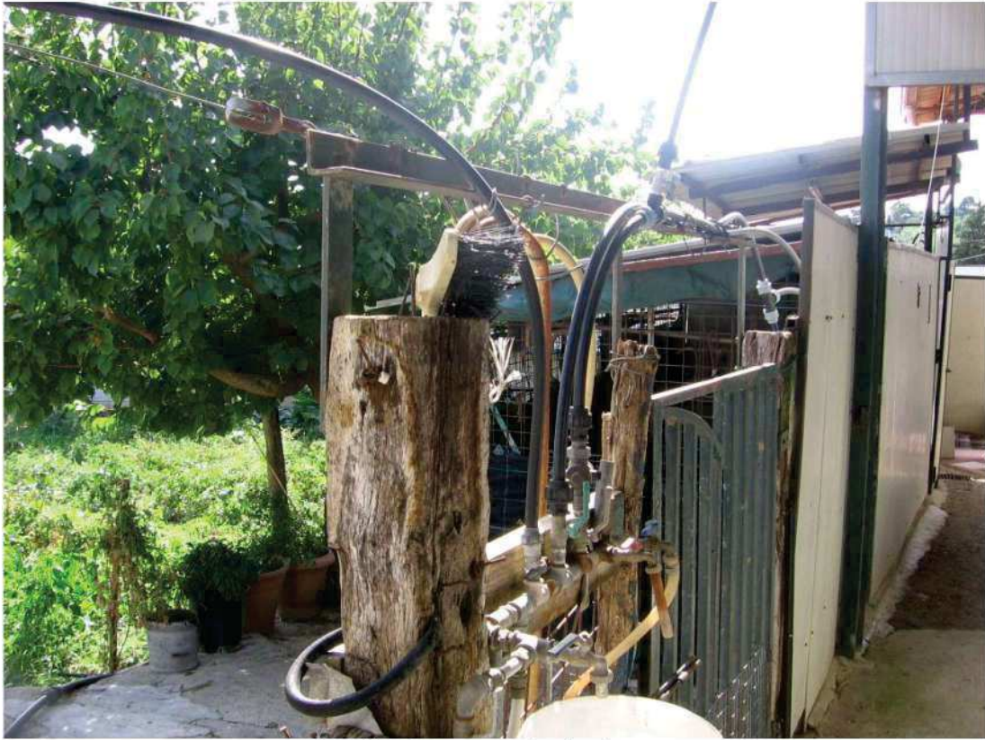
Strutture precarie abusive
