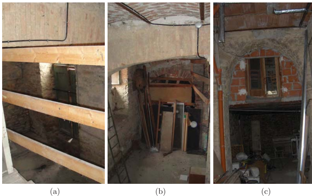
Figura 5: Locali cantine al piano seminterrato (a), (b) (c).
