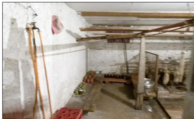
Piano terra – cantina
