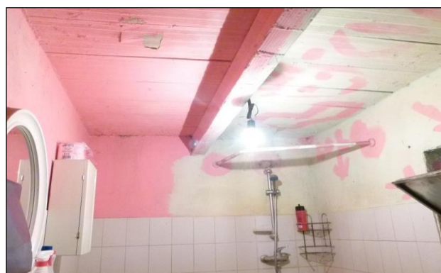
Piano terra – bagno
